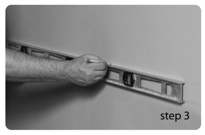
Use the level to draw a level line connecting the marks just made on the wall.
