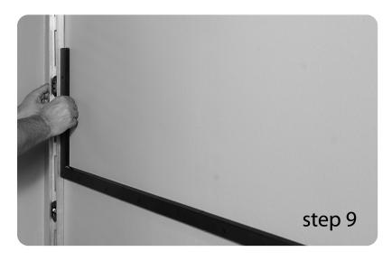
Attach corner sensor "L-B" to Sensor 9A to begin building upward (use level). Attach sensor 1A upward from left bottom corner piece and continue with sensors 2A - 3A. Then attach half-sized sensor piece 4A.
