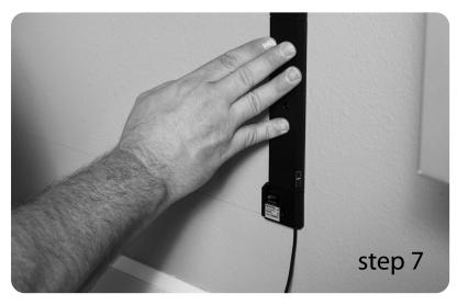
Return to bottom right hand corner on level line and begin build upward (Sensors 1- 3). Note the sensor number label located on the side of each sensor. Refer to the Installation Layout on Page 6 of this manual.
