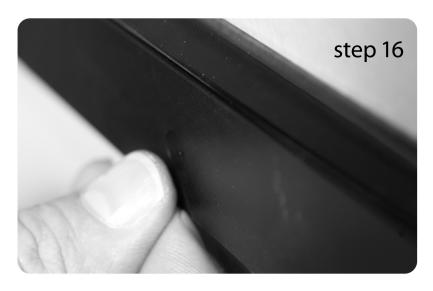
Once you have installed all the screws, push in the black plastic screw caps to cover the all the screws to create a nice looking install.
