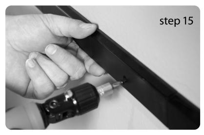
If you desired to make your installation permanent, screw in the black anodized screws.
