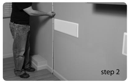
Select wall/whiteboard surface to mount WB80. The WB80 requires a 67.75" wide x 48.375" wide area. IMPORTANT: The wall must be flat to ensure the white board sensors have line-of-sight to each other. The wall can be slightly concave, but should not have any large bumps that could disrupt the path between the sensors. Use a level to ensure there are no such bumps.
