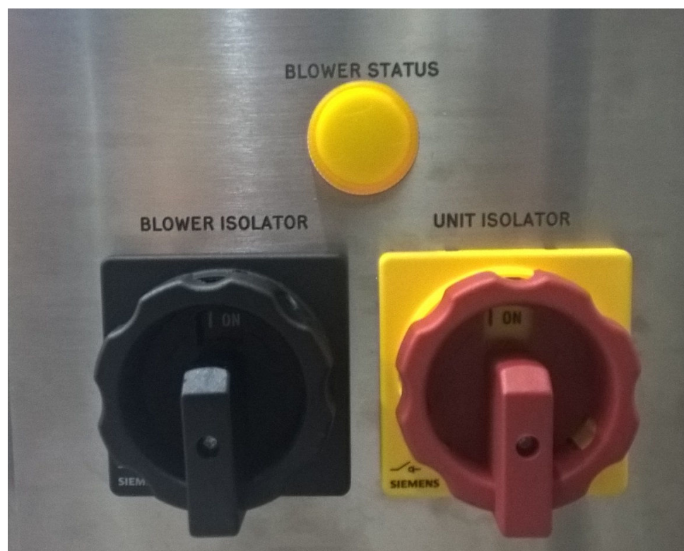
Figure 4-1: Isolation Switches
