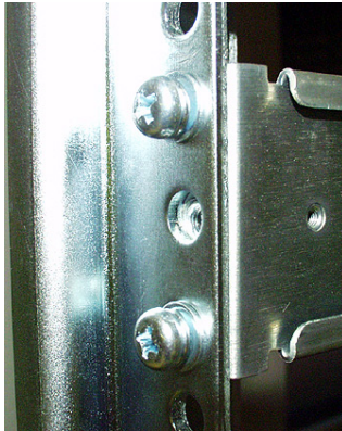
DS-16M Round-Hole Channel, Rack Front (for example, the CLARiiON Rack/Cabinet)
