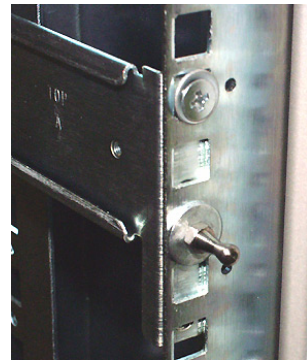
DS-32M Square-Hole Channel, Rack/Cabinet Front
