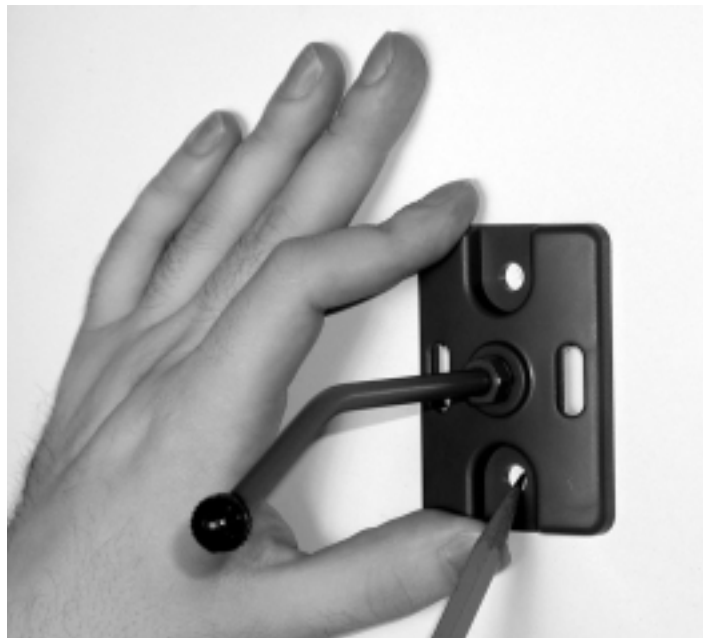
Figure 10 – Marking the Wall with the InvisiBall Base
