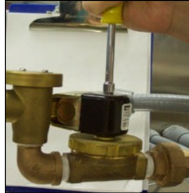
Removing the top screw
