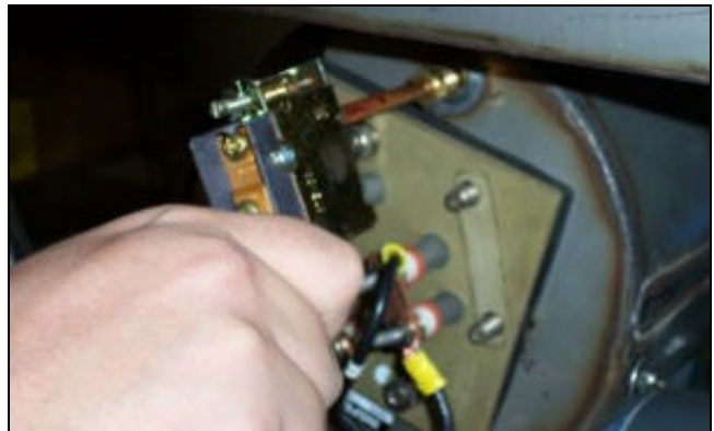
Putting the new thermostat in the well.
