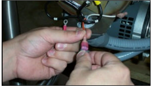
Attaching the jumper wires.
