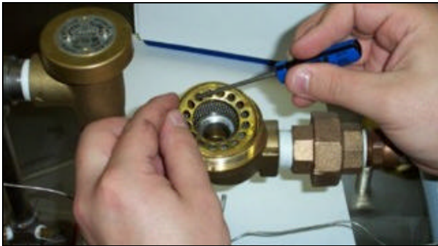
Removing the screen retainer
