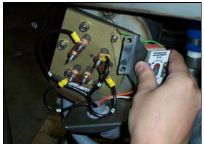
Removing the thermostat bracket.
