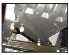
STEP 6 From underneath the enclosure, start the hardware through the holes in the bracket installed in STEP 2.
