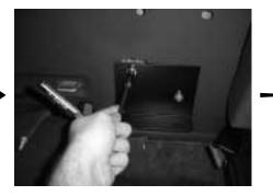
**STEP 5:** With the supplied hardware, attach the bracket to the rear wall.
