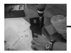
**STEP 19:** With a drill and 1/2" drill bit, drill holes at marked location of the washers.
