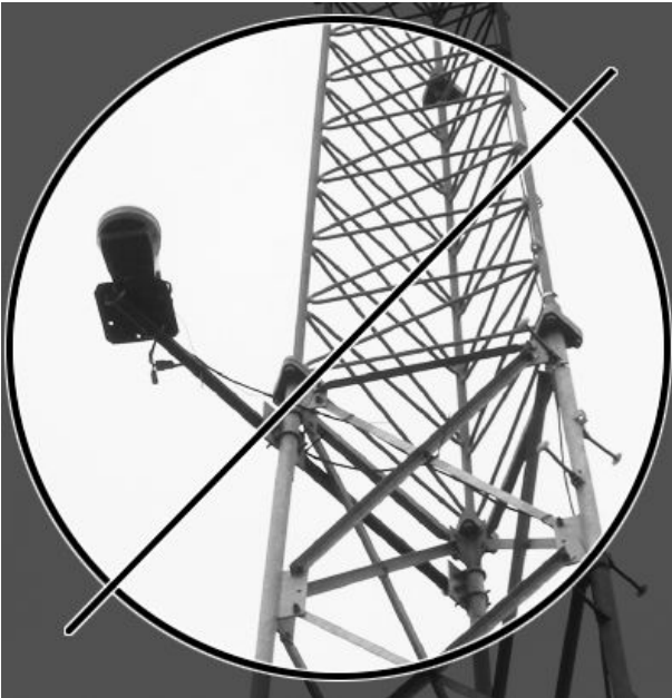
Receiver on Radio Tower
