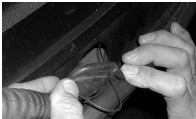
Figure 21: Entering the interior through the cable channel
