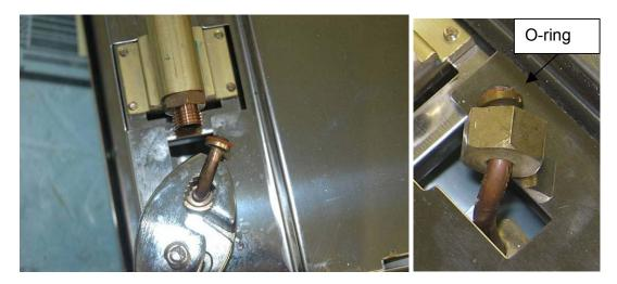
Tighten copper line connection. Do not over tighten.
