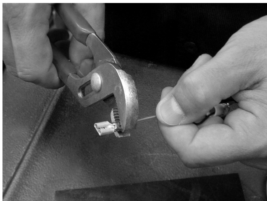
Attach appropriate connectors to wire leads.
