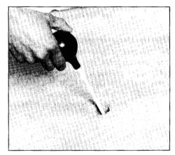
Put a plug on the anchor and hammer it into the concrete.
