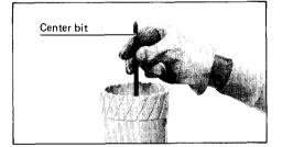
Rest the core bit on the concrete and turn the tool on. Once the core bit has cut a shallow groove into the concrete, remove the center bit. Then resume drilling.
