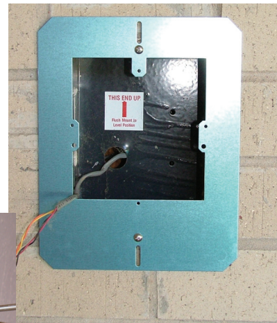
Figure 6 - DMCFR installation
