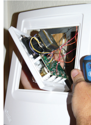
Figure 8 - Placing Room Station in
