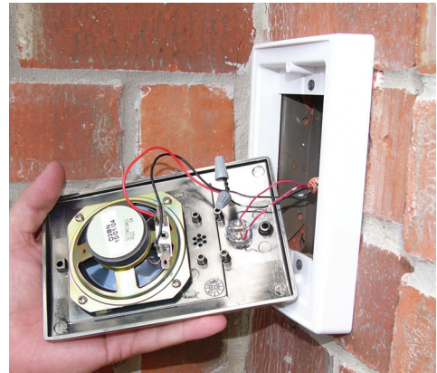
Figure 9 - DMCFD and Door Station Installation
