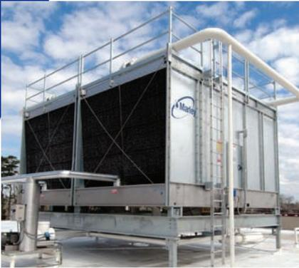
**Marley NC<sup>®</sup> Class Cooling Tower**—The flagship product of the Marley Package line comes with the most available options. Factory assembly is standard and the NC is available in galvanized or stainless steel. Cells available from 99 to 1,300 tons per cell. Factory Mutual Approval standard on most models and available on all models. CTI Certified.
