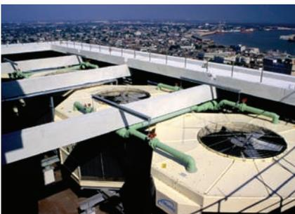
**Marley QuadraFlow<sup>®</sup> Cooling Tower**—Induced-draft, low profile design. These fiberglass and stainless steel towers are field assembled to facilitate siting, and are available from 129 to 1,047 tons per cell. CTI Certified.
