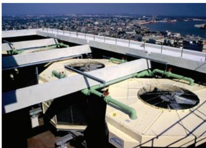
**Marley QuadraFlow® Cooling Tower**—Induced-draft, low profile design. These fiberglass and stainless steel towers are field assembled to facilitate siting, and are available from 129 to 1,047 tons per cell. CTI Certified.
