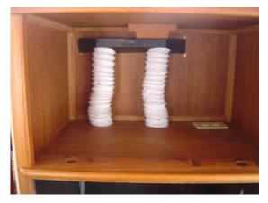
We drilled two 3 inch diameter holes in the back of the microwave shelf as well as an exit vent in the back of the microwave area.
