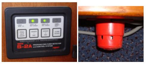
The Xintex/Fireboy S-2A we have can monitor two sensors, but only had one installed (the red thing in the photo above) under the galley drawers.
