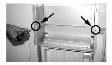
5. Pull forward on the extension plate to disengage the pins from the top channel stops, then slide it down into the inverter and push back to engage the pins on the bottom channel stops.
