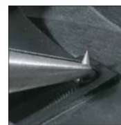
Replacing the discharger electrodes
