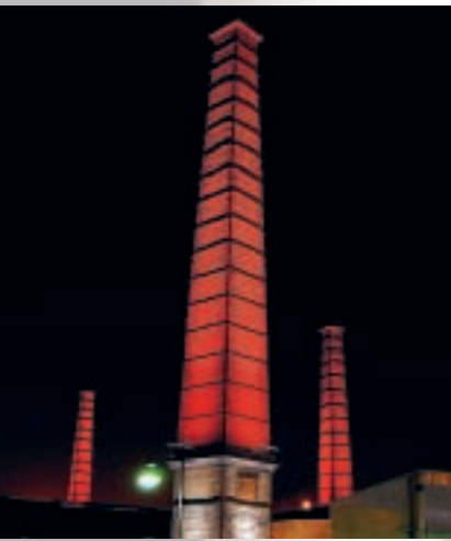
With an output of 60W of red Luxeons the chimneys of Technopolis, Athens, Greece, are visible from 1 kilometer. Lighting by Philips Luminaires.
