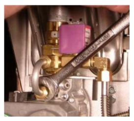
e. Thread the compression nut on the corrugated tubing end of the SCBS Valve Assembly onto the orifice assembly that you inserted into the runner tube in step c and tighten with a 1/2" (13 mm) wrench.
