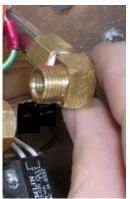
d. Mount the SCBS Valve Assembly into the appliance by loosely attaching the U tube end of the assembly onto the straight fitting that you installed into the TOP (Outlet Side) of the gas valve in step b.
