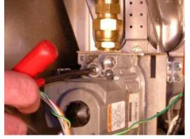
NOTE: CE approved models will have a pressure test fitting in this location. For CE approved models, remove this pressure test fitting using a 7/16" (12 mm) wrench. Using a 3/16" (5 mm) hex key, remove the plug from the auxiliary pressure tap on the manifold inlet and replace it with pressure tap fitting that you removed from the TOP (Outlet side) of the valve. Use teflon tape or apply pipe joint compound on the threads of the fitting to ensure a gas-tight seal.
