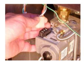
b. If your appliance has a solid-state control (or auxiliary thermostat) behind the door, remove it at this time. With a 5/16" nut driver remove the two self-threading screws that mount the control to the appliance, disconnect the control harness and tuck it out of the way to avoid damaging the harness during this procedure. Be sure to store the control in a safe place to avoid accidental damage to it.
