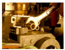
c. Remove the 1/8" NPT X 90° ¼" compression fitting from the other end of the SCBS Valve Assembly provided with the kit and install the orifice tip, also provided in the kit, on to the NPT end of the fitting. Insert the orifice end of this assembly into the runner tube installed previously in this procedure. **NOTE**: Check the orifice against the parts list included in these instructions to insure that it is the correct size for the gas type of your appliance.
