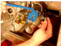
e. Using a 1 1/16" wrench and a 7/8" wrench, loosen the brass fitting on the top of the gas valve and disconnect the gas valve from the manifold inlet.
