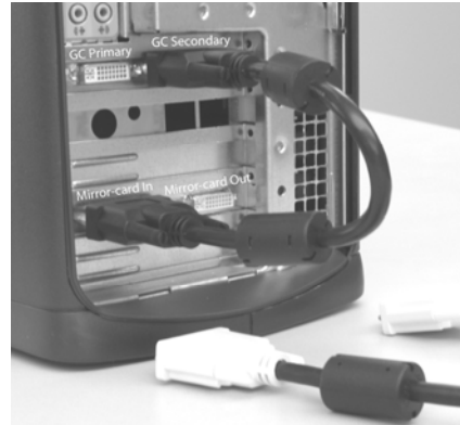
Short DVI cable installed
