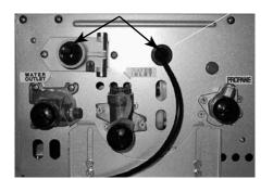
8) Connect the 4-pin connector from Communication Cable B to the 4-pin socket located at the top of the water heater control board of Unit 2. Communication Cable B ground wire terminal should be grounded with the PC board ground wire.
