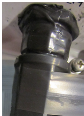
Figure 3.6. Wrapping the Connector with Rubber-splicing or Self-amalgamating Tape
