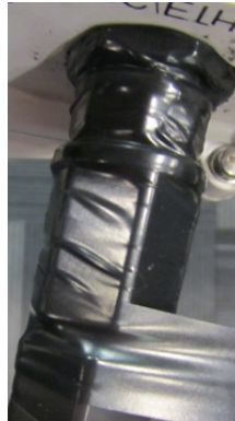
Figure 3.8. Wrapping the Connector with Electrical Tape
