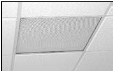
Figure 10: Completed subwoofer installation.
