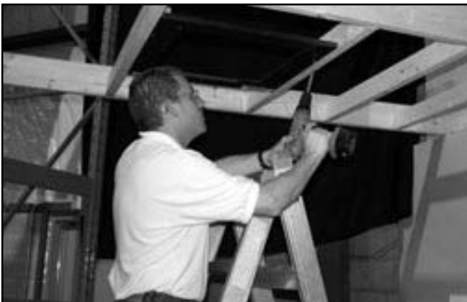
Figure 3: Attaching PIR to blocking.
