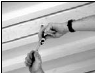
Figure 11: Installing the hanger bolt
