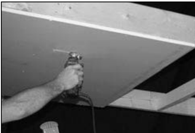
Figure 5: Cutting drywall using the Rotozip™.
