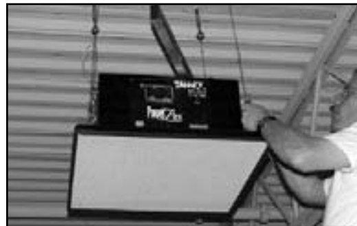
Figure 16: Leveling the subwoofer
