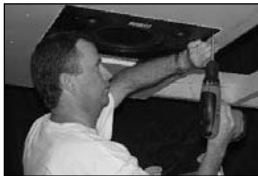
Figure 8: Attaching the subwoofer to the PIR.
