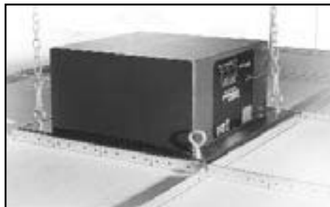
Figure 9: Installed subwoofer top view, only two chains attached
