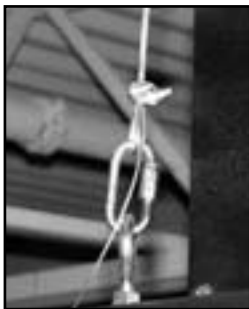
Figure 8: Wire rope detailing suspension or seismic tether
