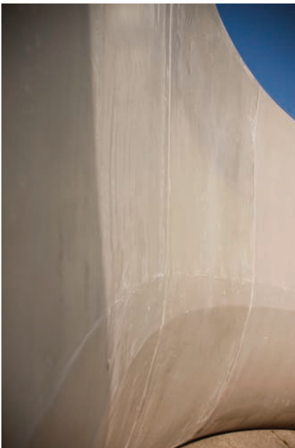
The RTM process has smooth texture on the interior as well as a smooth gel coat surface on the exterior
