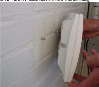
Figure 12 KIRK Wireless Server 600v3 Wall Mounting
