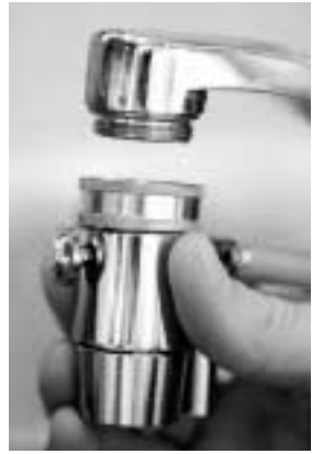
Figure 10 Attaching diverter to Faucet
