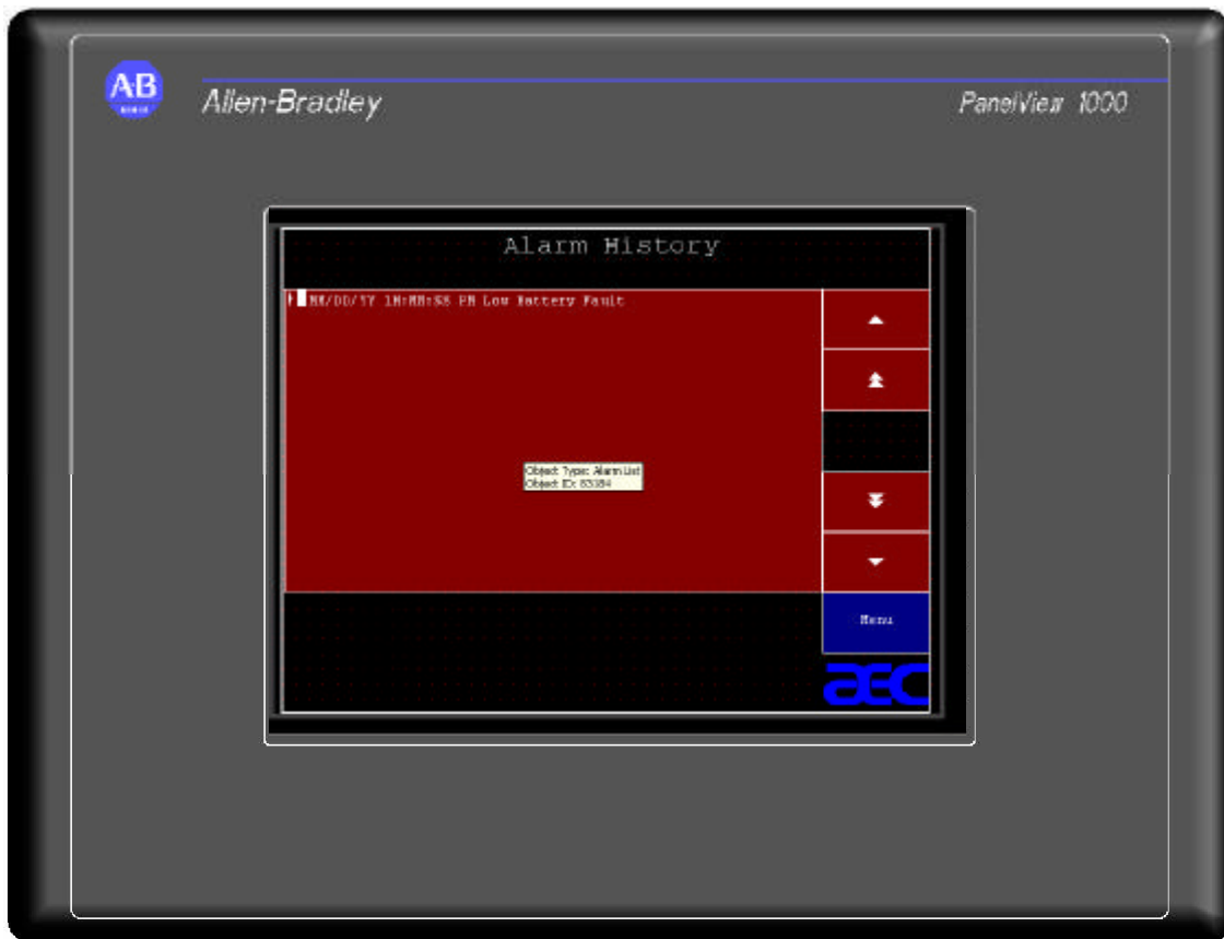
Figure 15 Alarm Condition Screen
