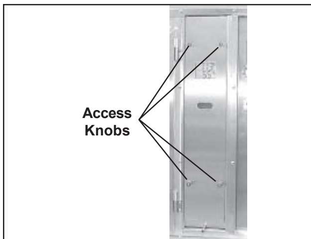
Figure 62. Filter/Fans Compartment Access Knobs
