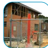
Prevent Building Site Theft
