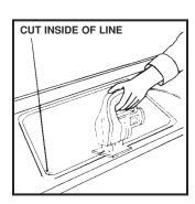
4. Using a saber saw, cut inside of cutout line. Trial fit sink to check proper fit.
