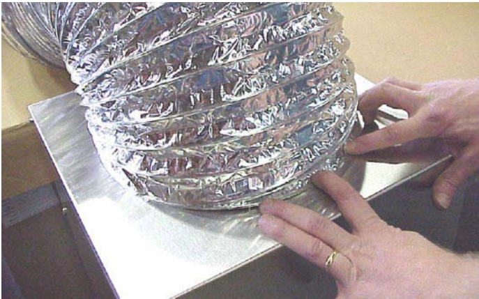
Figure 5: Inlet ducting
