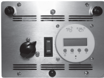
Item 1: Ventilation Timer & Humidity Control
