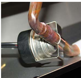
Figure 5: Defrost thermostat
