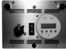
Figure 11: Ventilation Timer and Humidity Control Panel
