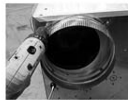
Figure 4: Installing exhaust collar.
