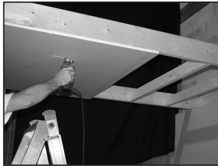
Fig. 5: Cutting drywall using the Rotozip™.
