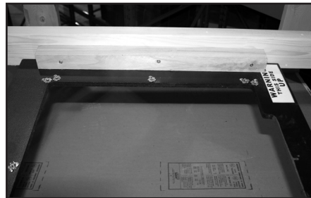
Fig. 2: Overhead view of pre-installation ring, showing blocking attached to joist.
