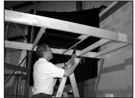
Fig. 3: Attaching pre-installation ring to blocking.
