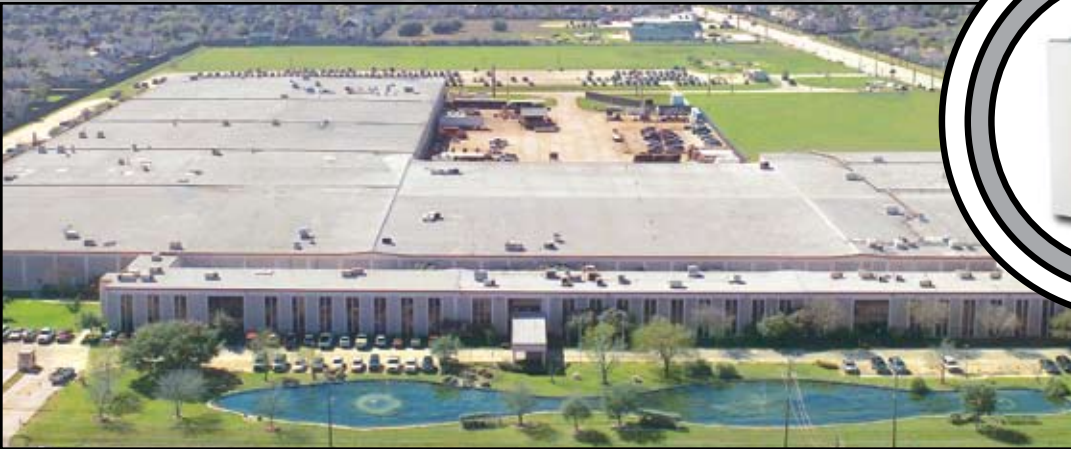
North American Headquarters & Manufacturing Facility (Houston, TX)
