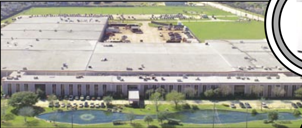
North America Headquarters & Manufacturing Facilities (Houston, TX)
