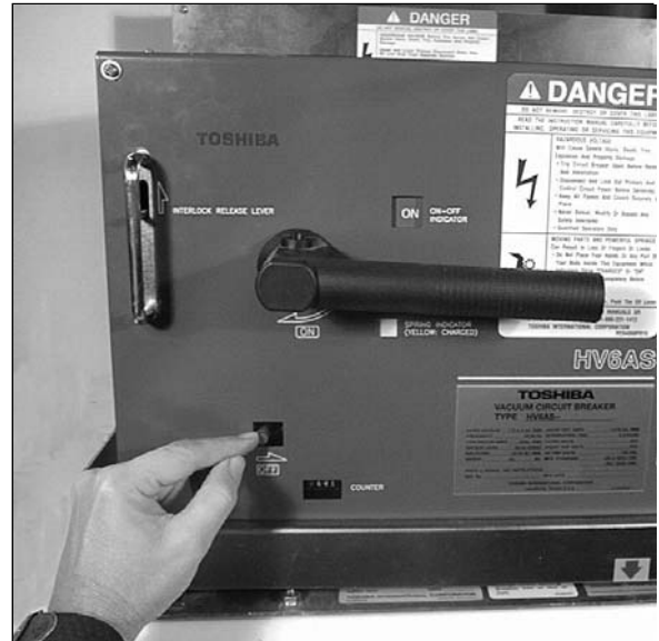
Fig. 27 Manually Opening Breaker
