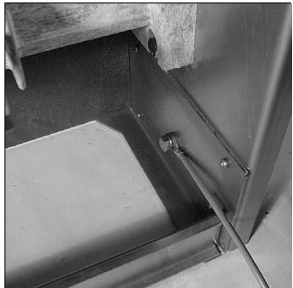
Fig. 14 Installation of Ground Wire
