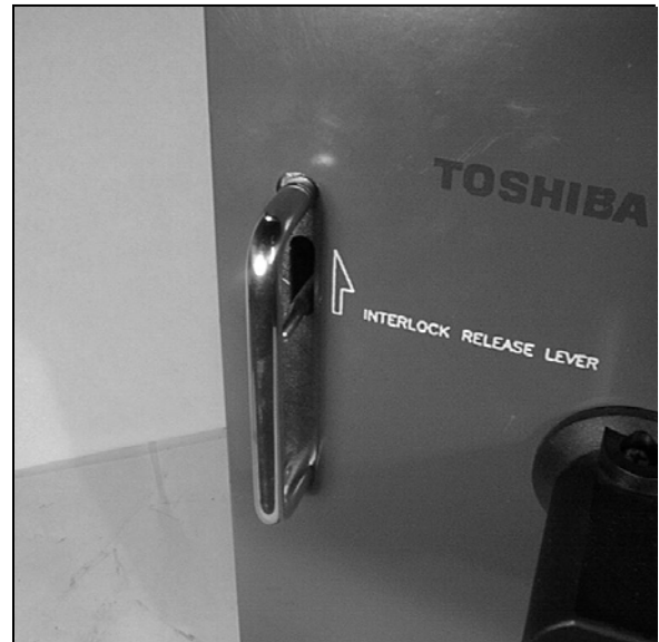
Fig. 3 Interlock Release Lever
