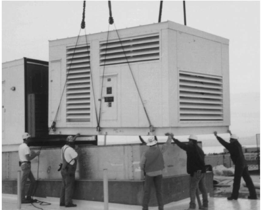
Figure 3. Use proper lifting and rigging methods
