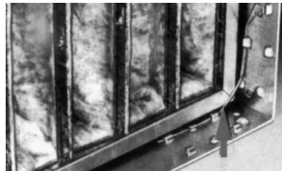
Figure 23. Bag filter show with C-70 fastener
