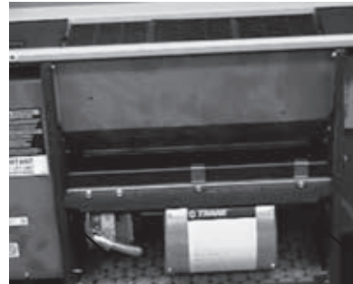
Figure 35. Remove the two mounting screws located under the fanboard to slide it out.
