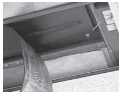
Figure 34. To remove the main drain pan on horizontal fan-coil units, peel the insulation from the edges of the pan's underside to access the mounting screws.
