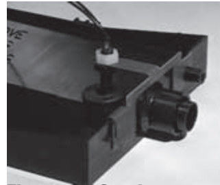
Figure 13. Condensate overflow switch installed in a horizontal auxiliary drain pan.
