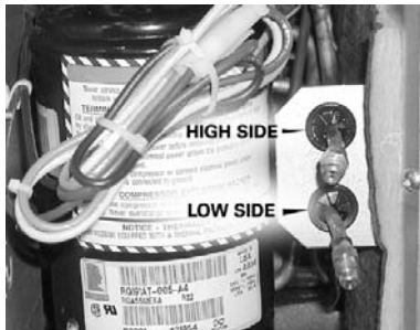
Figure 11: Schrader connections
