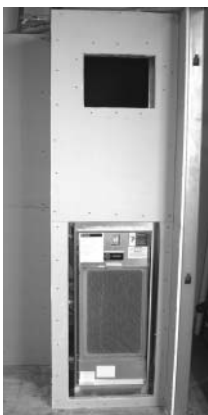
Figure 11: Install chassis centered
