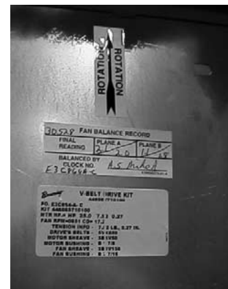
Figure O-M-4. Location of fan belt label on fan scroll.
