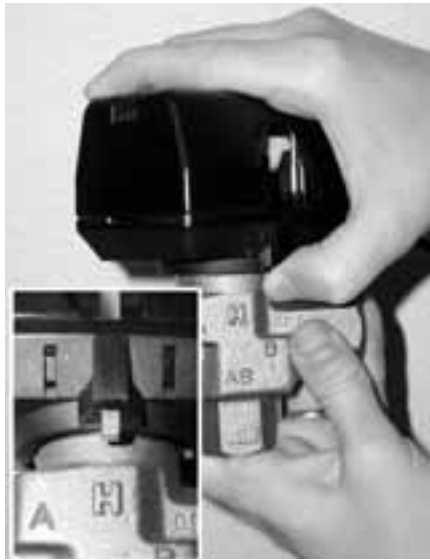
Figure 6a: Remove modulating valve actuator by pressing in tab (inset) and turning actuator 45° counterclockwise.
