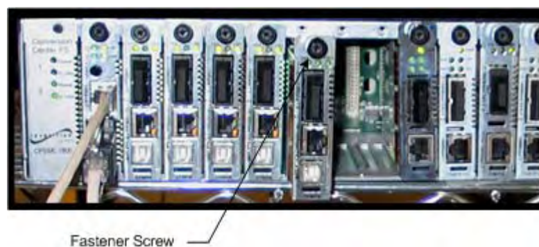
Figure 12: CFBRM/CBFFG Device Chassis Installation
