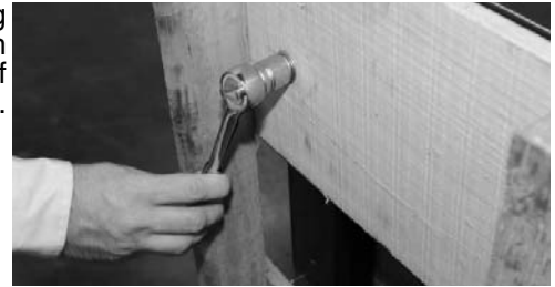
Removing skid from bottom of cabinet.
