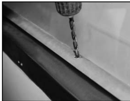
Image 3 (Drilling lock bracket hole)
