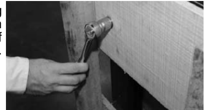
Removing skid from bottom of cabinet.
